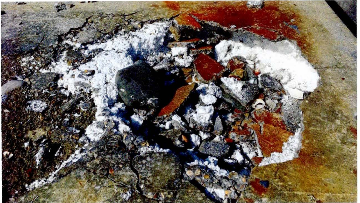
Figure 9: Erosion on the cement faced upper pontoon
